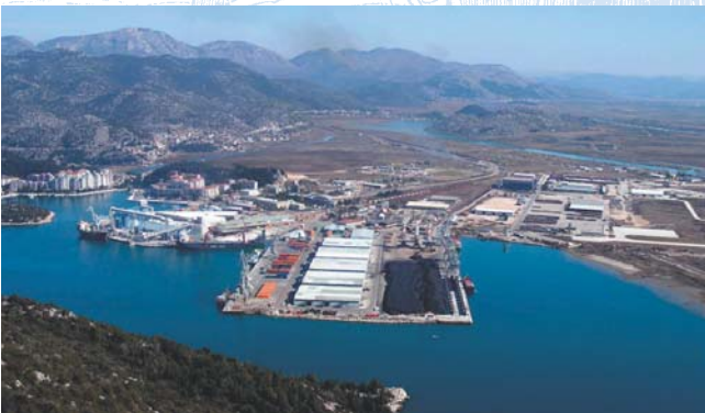
The Port of Ploče, the construction site of a large container terminal and bulk freight terminal
