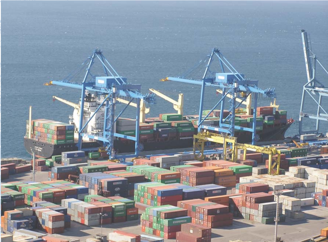
The »Brajdica« Container Terminal in Rijeka has seen a constant growth in container transport
